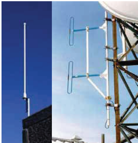
Omnidirectional (left) and offset dipoles (right) serve as data receptors for the dispatch control center
